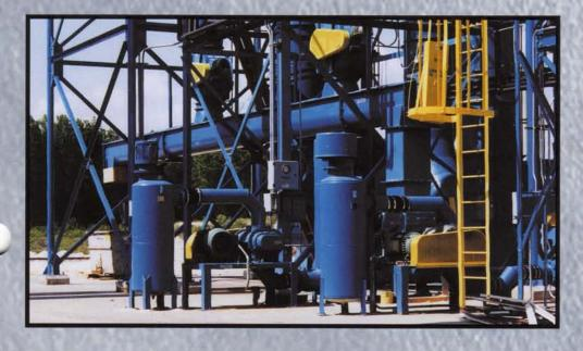
While Aircon baghouse tops may rise majestically above a dust-free skyline, an important part of the installation is in fact much closer to the ground. Heavy-duty structural steel supports can be built in varying heights to accommodate new and old roofs, ductwork, and high-pressure dust conveying lines. Especially noteworthy about this installation is its easy navigable stairway and ladder egress.
