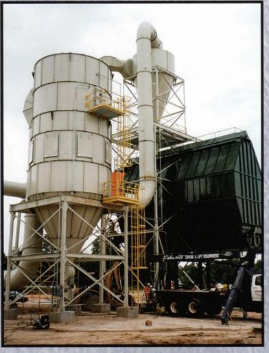
The Aircon baghouse and cyclone shown above were installed in a pine board plant. Dust is collected from one of the nation's highest capacity planers, operating over 1200 feet per minute.
