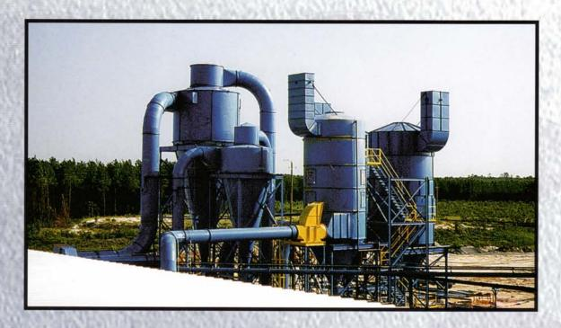
The presence of the big blue reverse air baghouses (above and opposite page) signals both the end of dust problems and the beginning of effective material recycling for this MDF facility. A smaller beige compressed air unit (lower right) stands above the silos of a particleboard plant.
